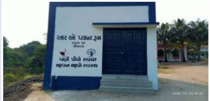
RO Room and RO with Chilling unit at village Charetha, Taluka Mangrol, District Surat
