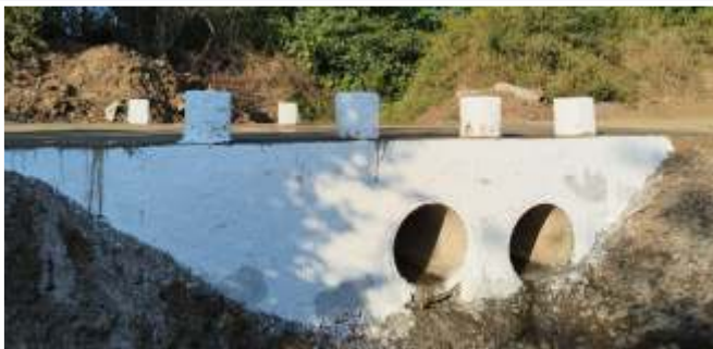
WBM Road with culverts at village Juna Bhaga, Taluka Valia, District Bharuch
