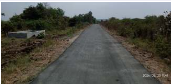
Asphalt Road at village Shah-Charetha, Taluka Mangrol, District Surat
